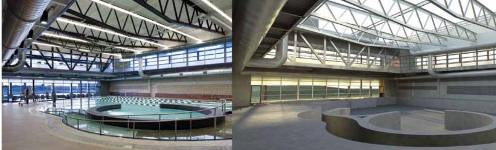
These images of the natatorium as-built (left) and the BIM (right) illustrate the coordination of the complex architectural, mechanical, and structural systems afforded by using IPD.
