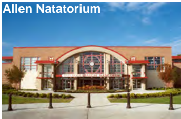
Allen Natatorium, Allen ISD, TX
